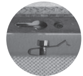
The head engages in the rail screwed to the ceiling
