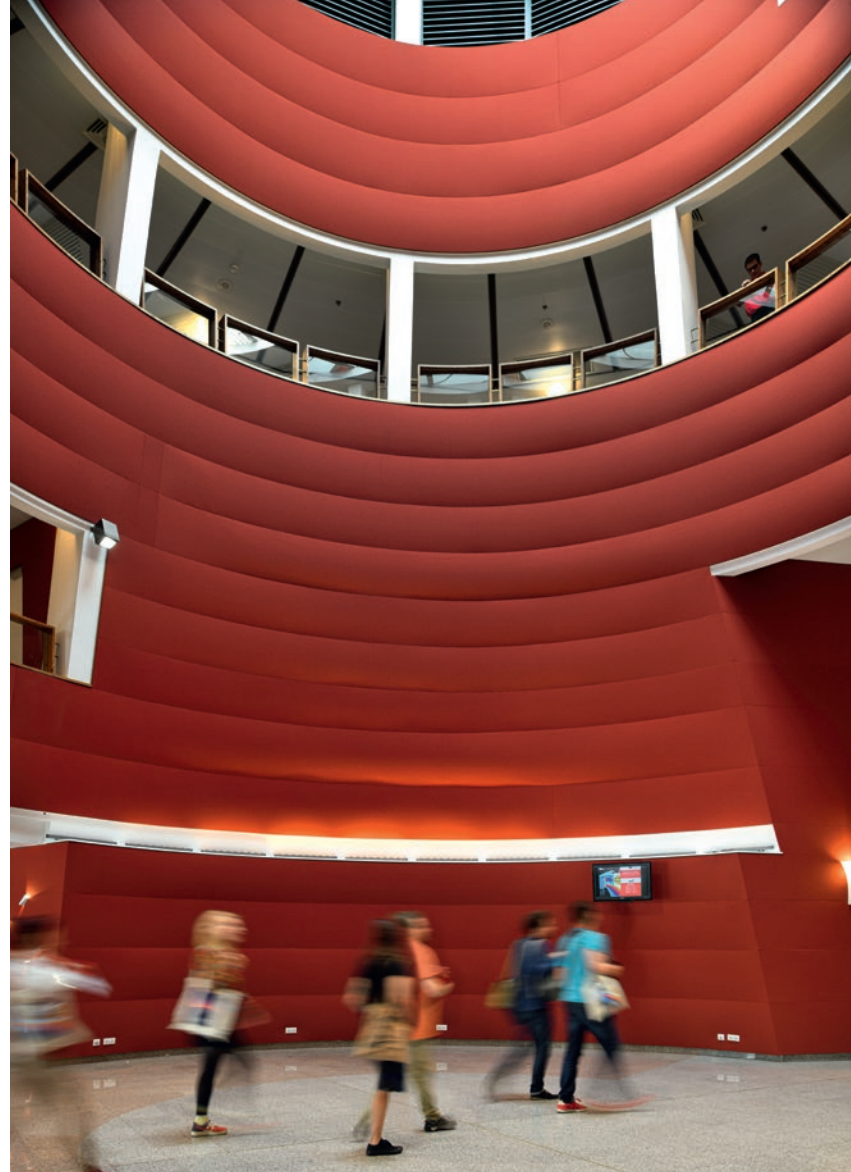
↑ → Vibrasto acoustic cladding fitted to a concave wall. The flexibility of the tensioning battens makes it possible to fit the shape. Polydome Congress Centre in Clermont-Ferrand in central France. Yves Bellaigues, Clermont-Ferrand city architect.
