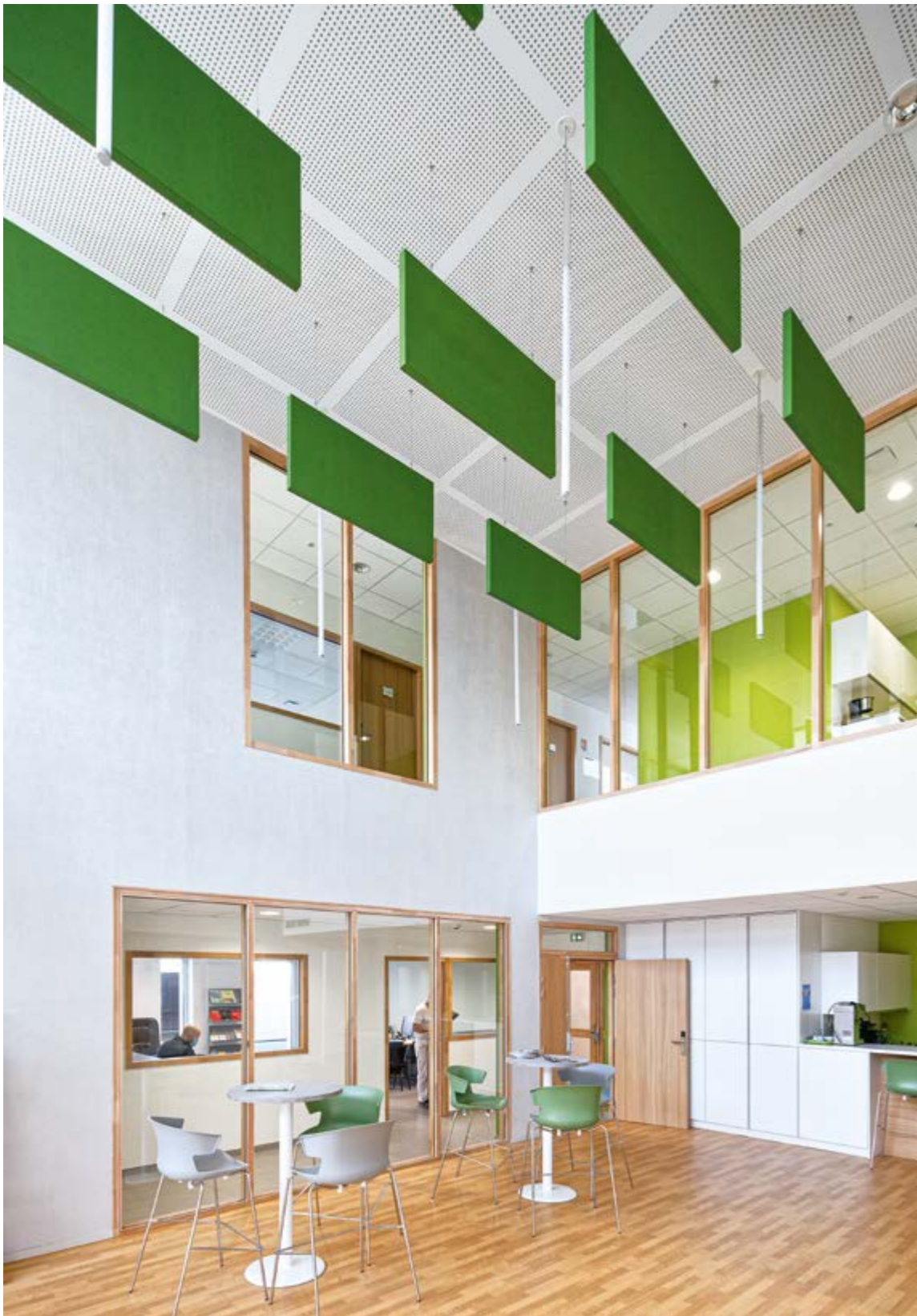
Stereo acoustic panels suspended from the ceiling as baffles in the administrative centre of Sevadec (Calais's waste removal and recycling operations). Polynome architectural workshop, 2020.
