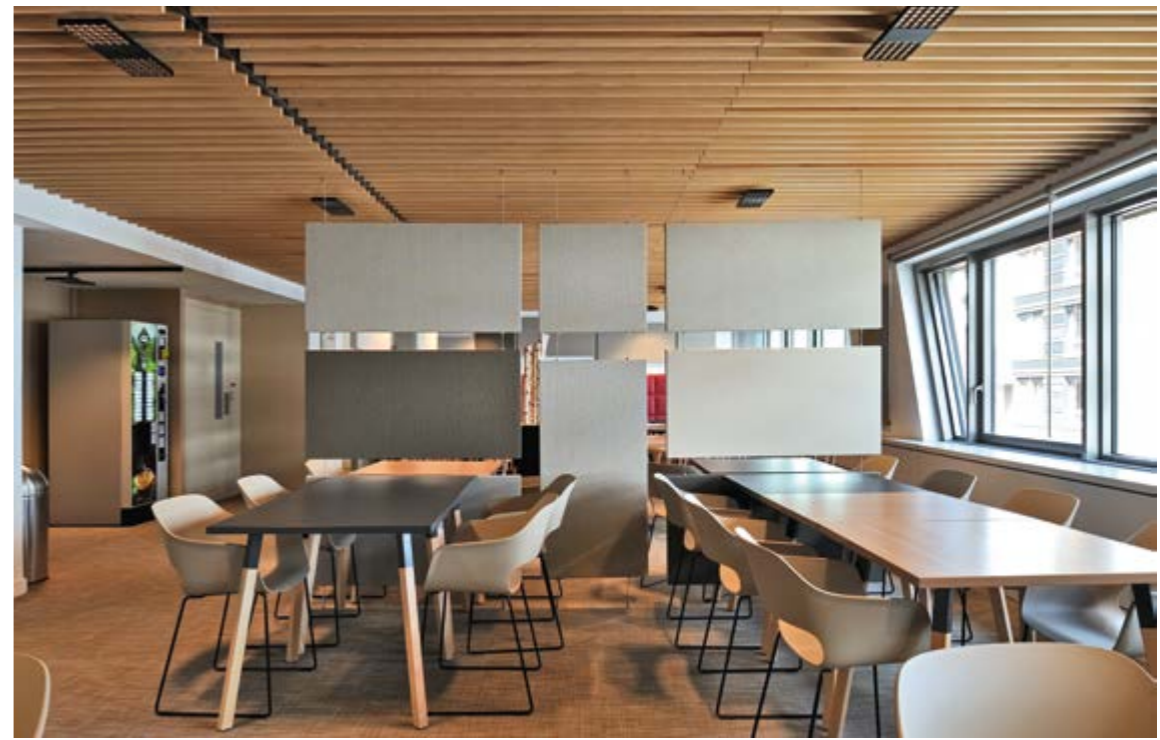
A partition of Stereo acoustic panels suspended from the ceiling on cables that run through them and are anchored to the floor in the head offices of the regional authority in Lyon Confluence FERRAND-SIGAL Architectes & Associés. Acoustics by EAI, 2022.
