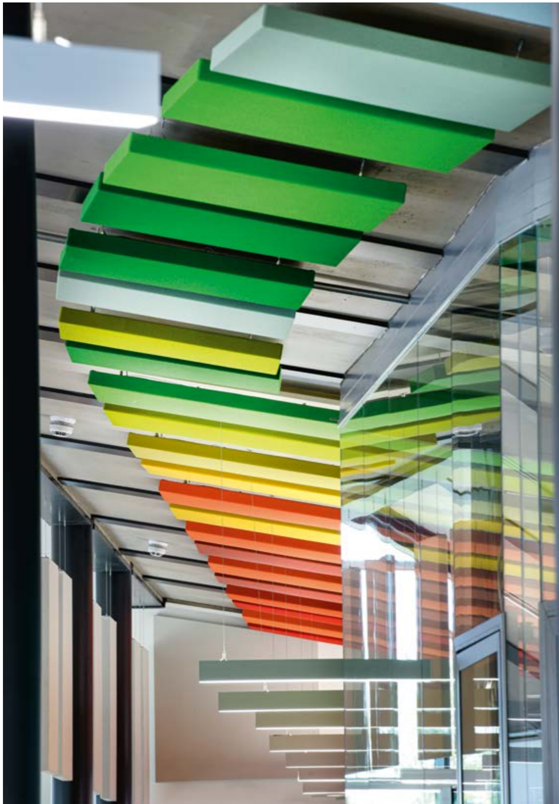
Stereo acoustic panels suspended from the ceiling of the office area of the Royal Horticultural Society in Wisley, UK. Geoff Turner, associate Director of WilkinsonEyre, 2021.
