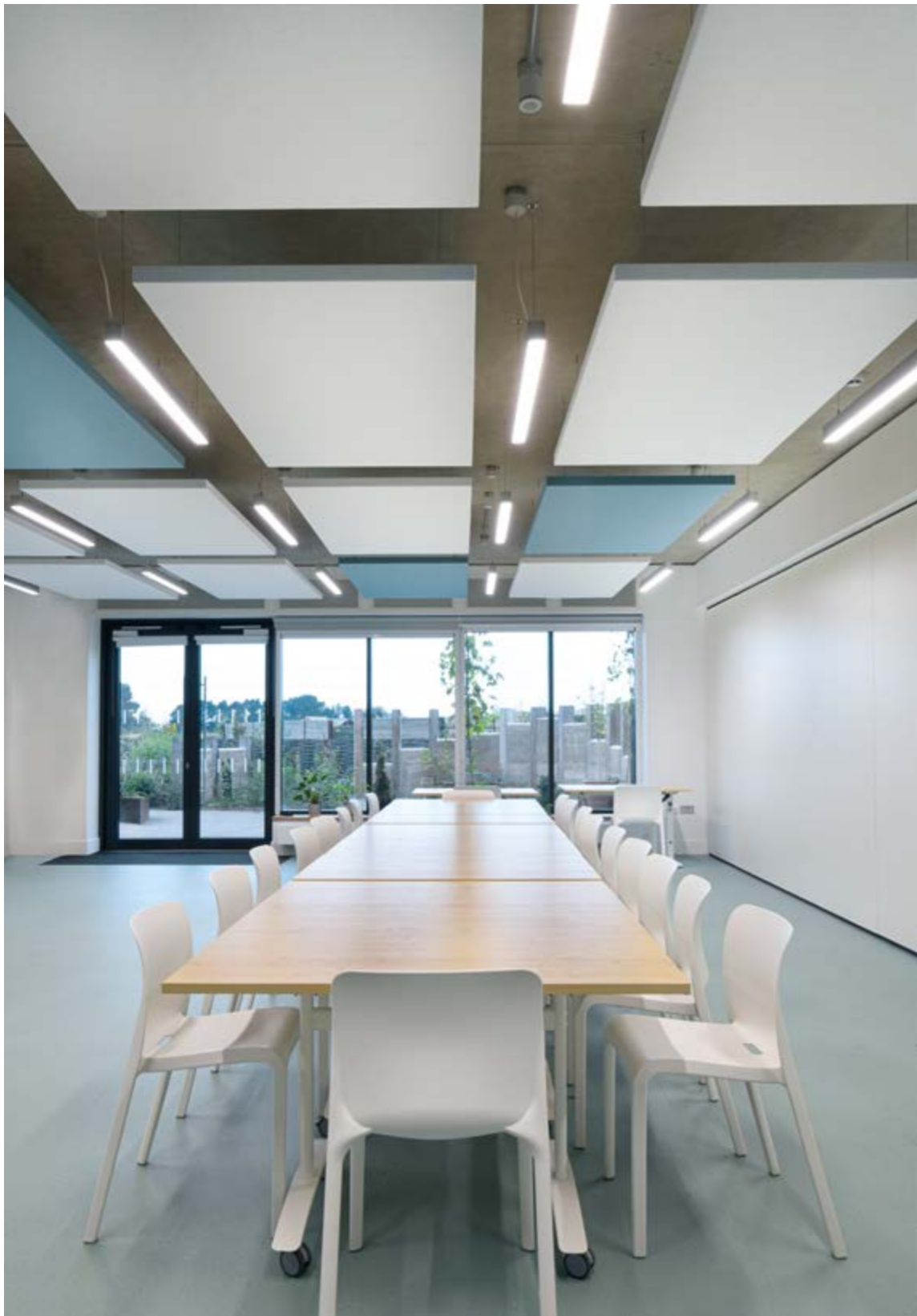
Stereo acoustic panels suspended from the ceiling alternating with lighting in classrooms at the Royal Horticultural Society in Wisley, UK. Geoff Turner, associate Director of WilkinsonEyre, 2021.
