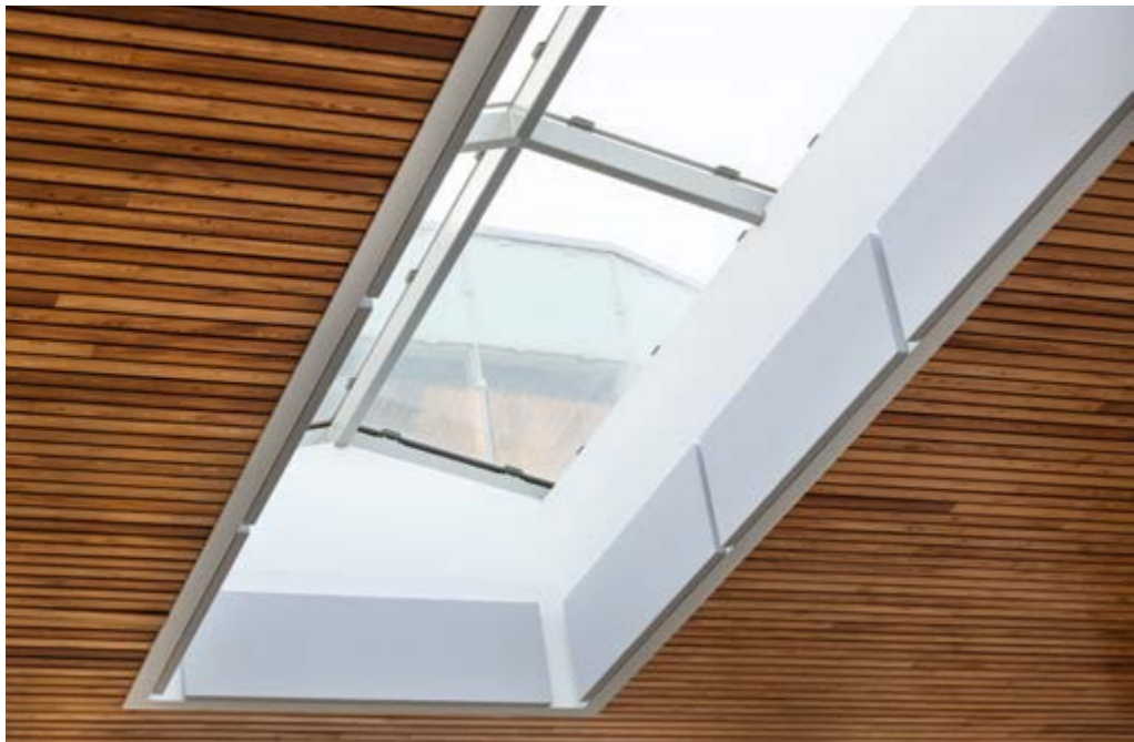
Worcestershire Park Railway Station in UK. Architect: Mark Alton of Mott MacDonald, 2021.
