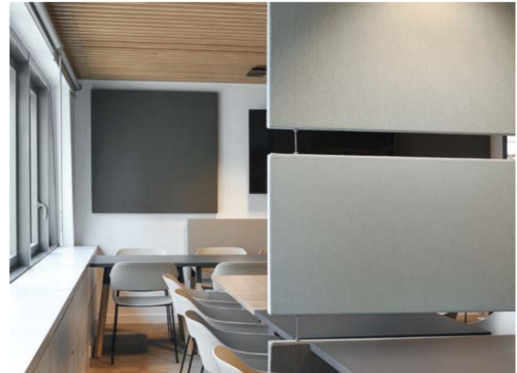
A partition of Stereo acoustic panels suspended from the ceiling on cables that run through them, and Stereo acoustic panels fixed to the wall using magnetic fixtures, in the head offices of the regional authority in Lyon Confluence. FERRAND-SIGAL Architectes & Associés. Acoustics by EAI, 2022.
