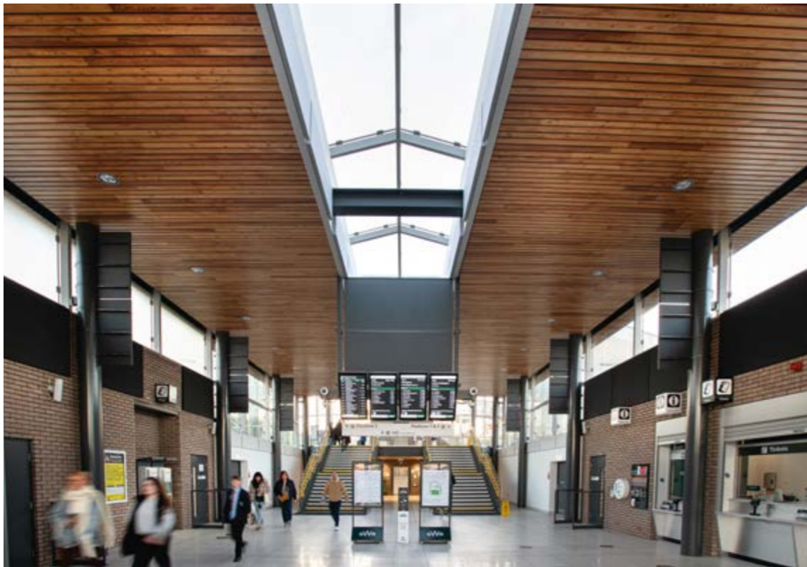
Stereo acoustic panels fixed to the wall in Worcesterstershire Park Railway Station in UK. Architect: Mark Alton of Mott MacDonald, 2021.
